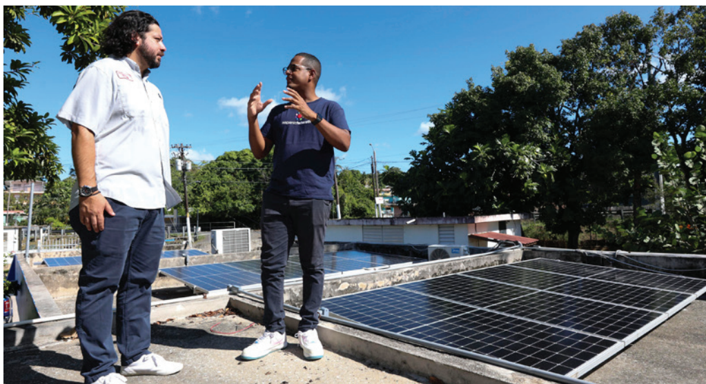
▲ HF staff and partner during solar panel installation, Cabo Rojo, PR
